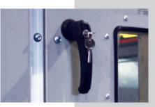
Handles are a thermal bridge issue. Hands can get scraped with door handle. External handle mounted on unit casing.
