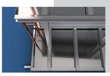
**Cascading auxiliary drain** connections can cause the lower auxiliary drain pan to overflow.
