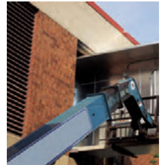
Air Handler Replacements
