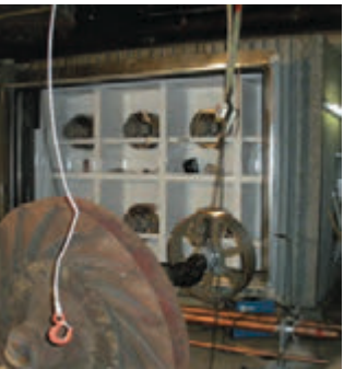
Fan and Coil Replacements
