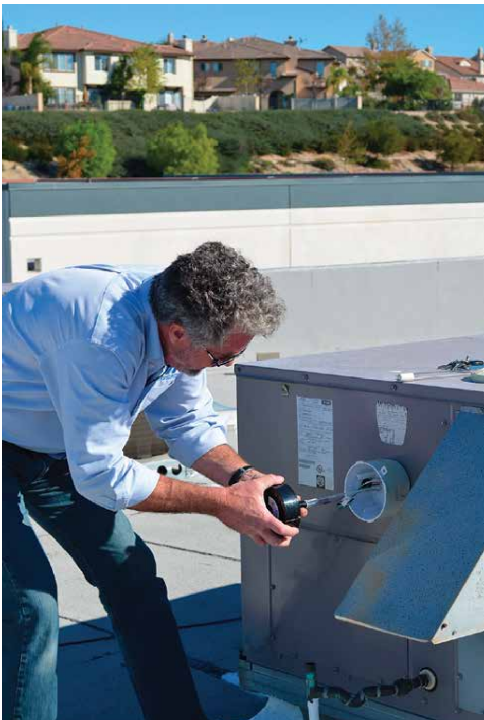
The economical, X-Plus extended UV-C Lamp-base fixture from UV Resources can be easily mounted from the exterior of any HVAC system, making it ideal for hard-to-access outdoor and indoor equipment up to 30 tons.
