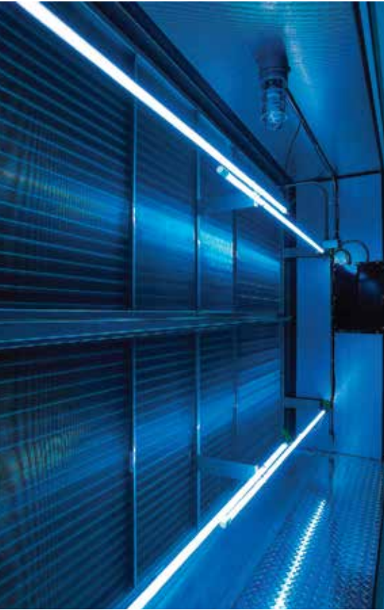
The RLM Xtreme fixtureless UV-C lamp system from UV Resources creates a more energy-efficient HVAC system that doesn't have to waste energy to move air.
